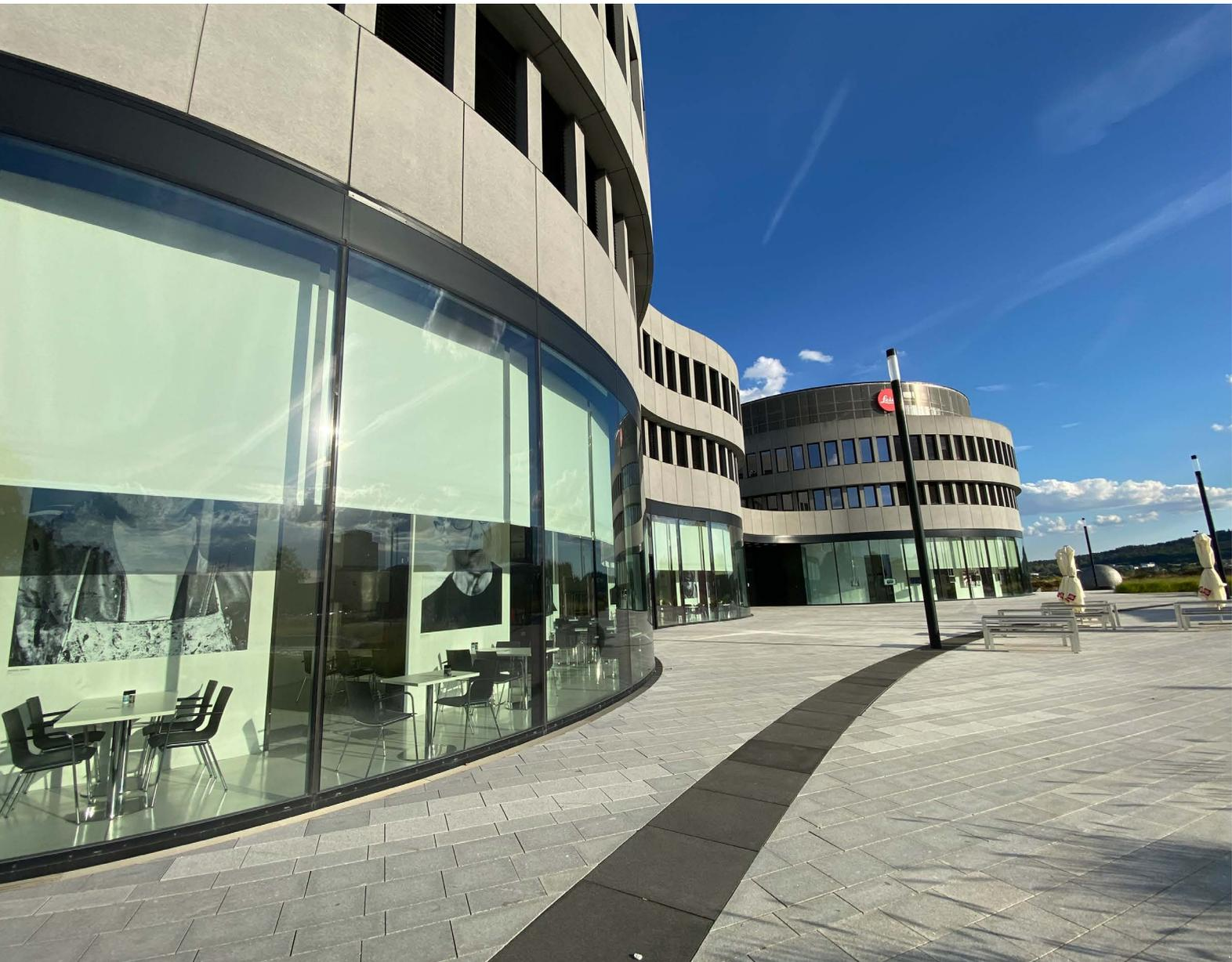
Leica Camera AG headquarters in Leitz Park resembles camera lenses. Designed by Gruber + Kleine-Kraneburg Architekten, the building has a 5-meter tall Guardian SunGuard SuperNeutral 70/41 curved glass facade that balances solar control, light transmission and thermal insulation.
